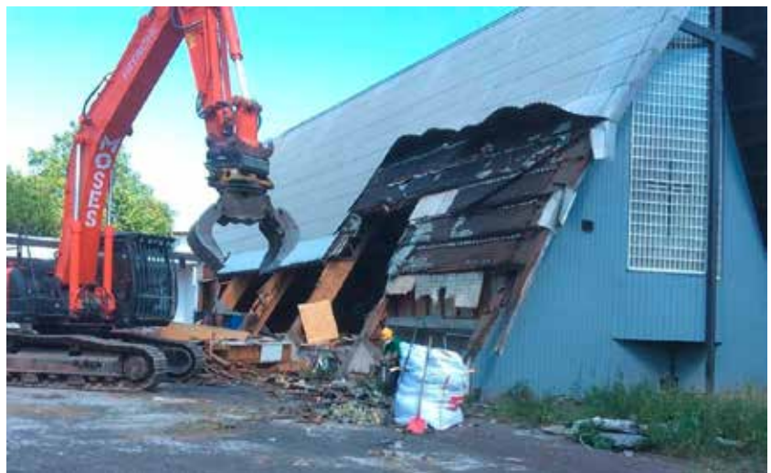
Bethel International Baptist Church building is demolished.
